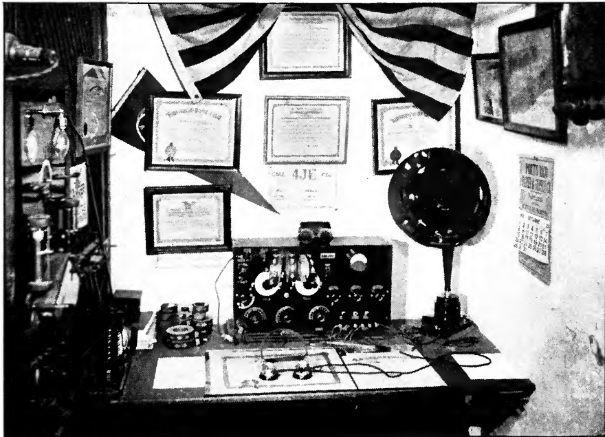
A PRE-WAR MULTI-RANGE RECEIVER Designed for transatlantic work with a single tube
